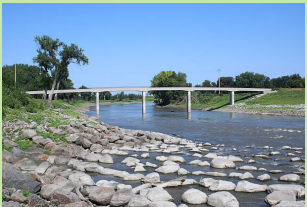
Partially modified: e. g. foot consolidation with boulders
